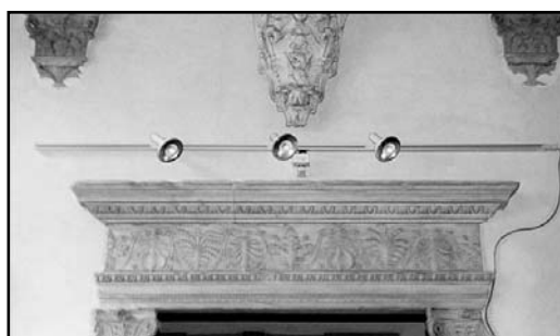
New luminaries installed
