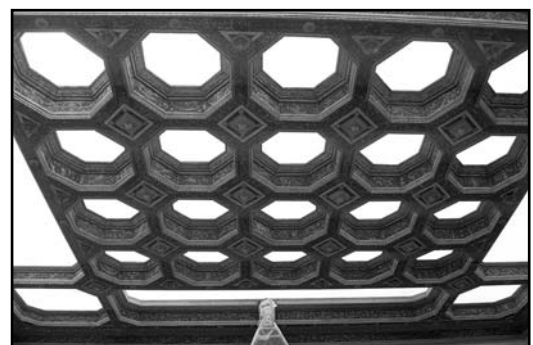
The diffuser panels installed on the old wood ceiling
