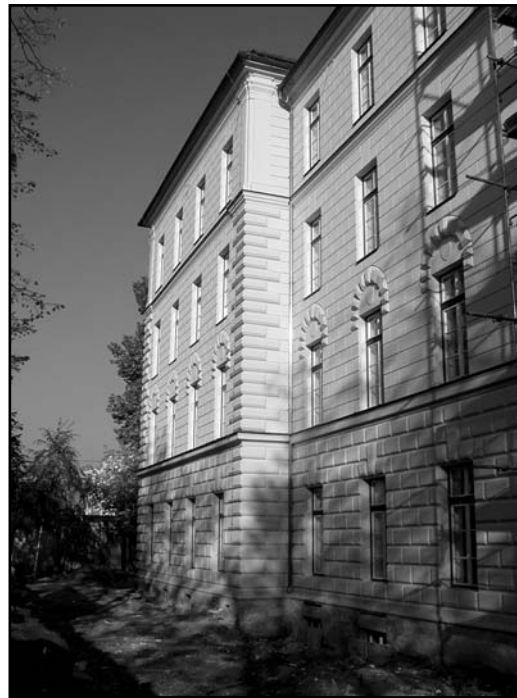
Refurbished part of the building after the renovation
