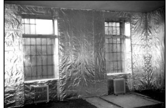
Preliminary testing and monitoring, reference room, 2nd floor
