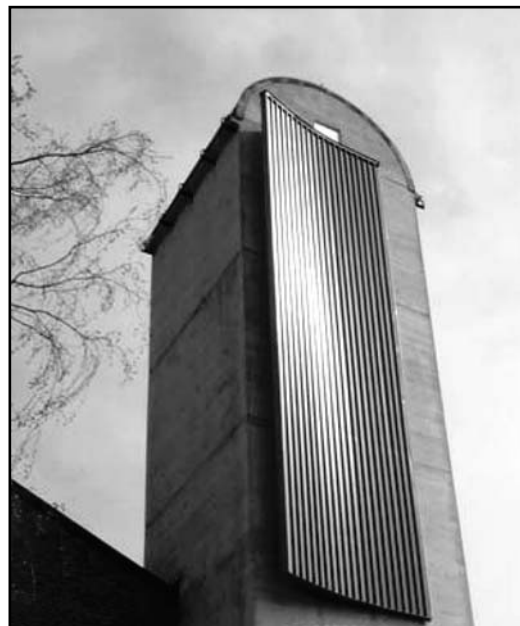
Solar air collector installed to the charcoal tower
