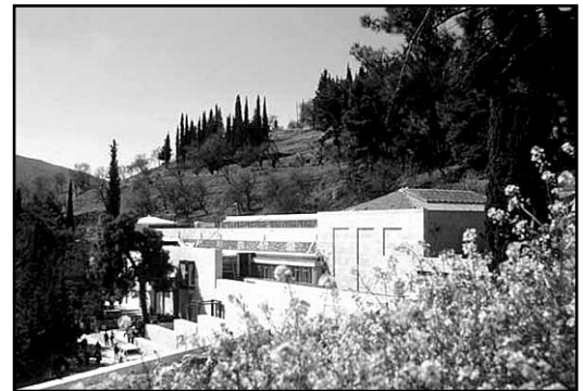
The Archaeological Museum of Delphi is built of both durable and traditional materials which guarantee long life and low maintenance costs
