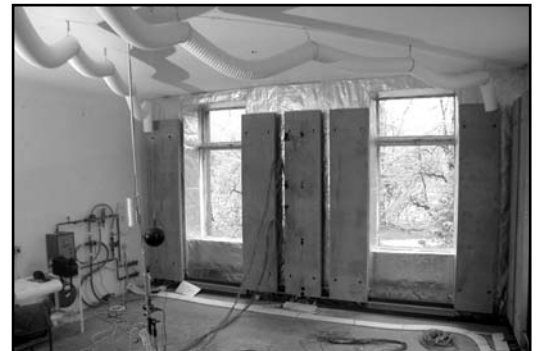
Preliminary testing and monitoring, model room, 1st floor
