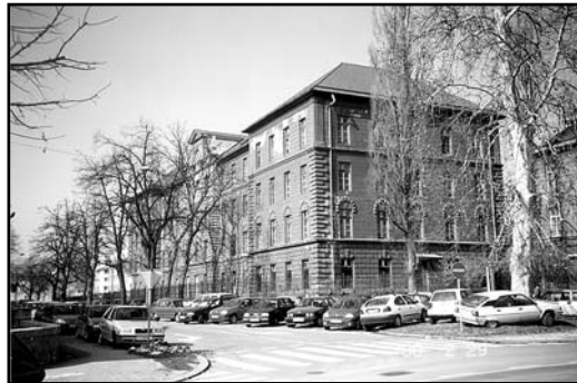
Building of SEM before reconstruction, south-east view
