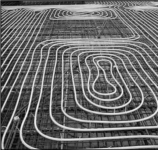
Ceiling with a system of plastic tubes for concrete core heat storage
