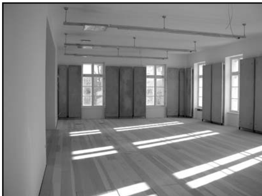
Refurbished interior view with heating-cooling panels and example of sun patches study
