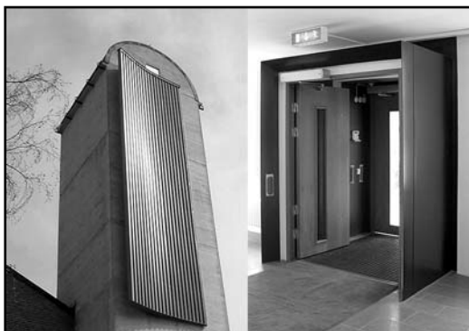
An air-lock has been built at the main entrance
