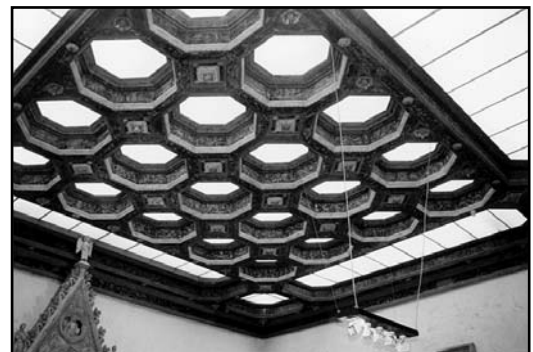
The existing skylight: internal view
