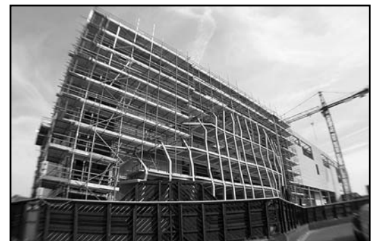
THEpUBLIC Arts Centre (under construction)
