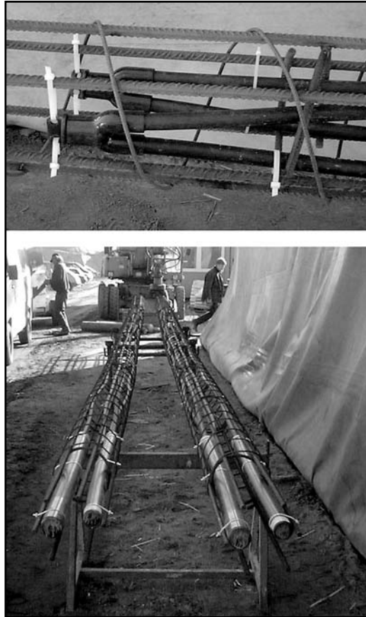
Reinforcement and U-tubes of energy piles
