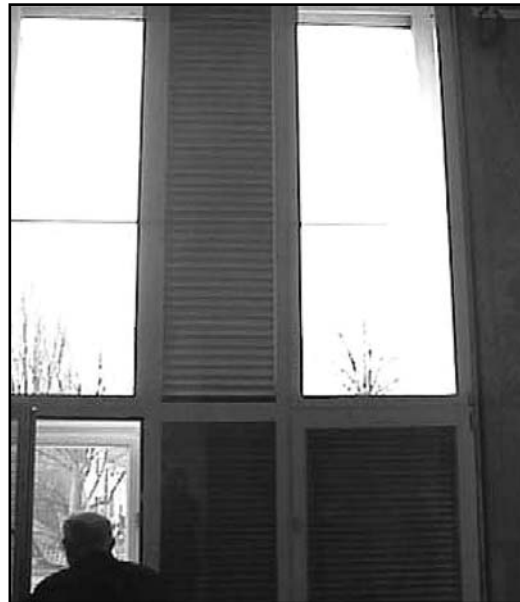
Two-part louvre blinds during installation at Herzog-Anton-Ulrich Museum
