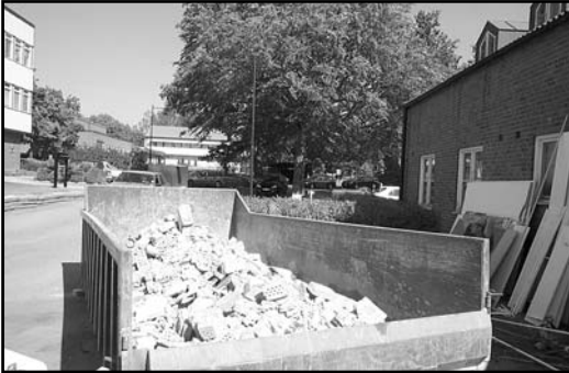
Building waste is sorted at the building site in the Kristinehamn Museum of Contemporary Art project
