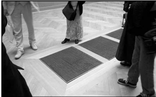
Existing natural ventilation systems in Herzog-Anton-Ulrich, Braunschweig. Above: Air inlet integrated in the floor. Below: Skylights for daylighting and extraction of used air
