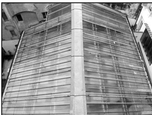
The existing skylight: external view
