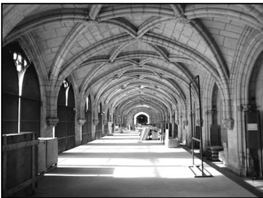
Ground floor view
